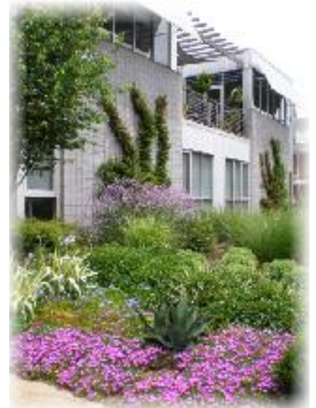
This office complex and gardens have been designed to work together in harmony with the environment.
